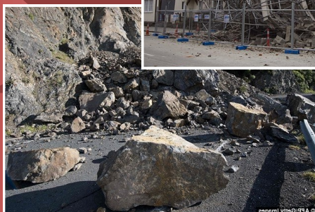
Some of the earthquake damage.
